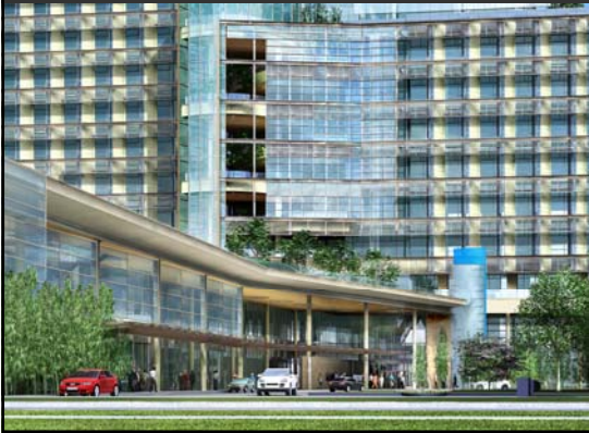
PMC West - Exterior View
