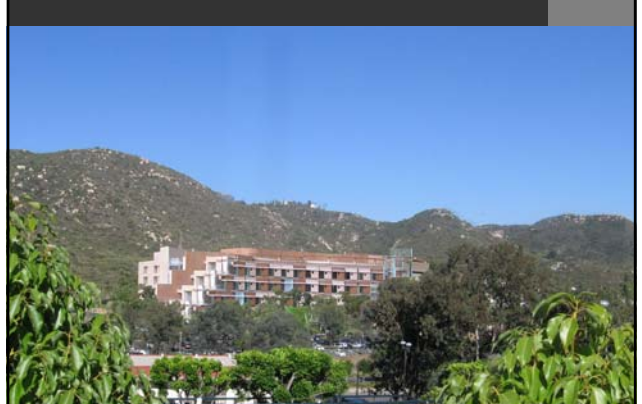
Pomerado Hospital - Exterior View
